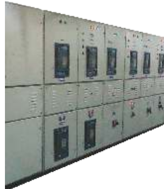
PCC Panel (Power Control Center Panel)
