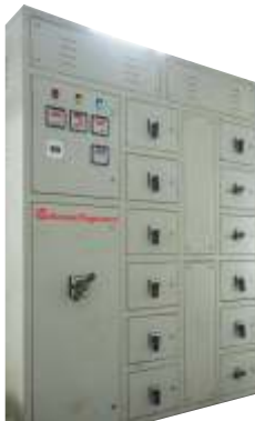
MCC Panel (Motor Control Center)
